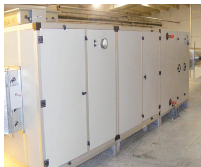
Installation of a Chilled Water AHU
