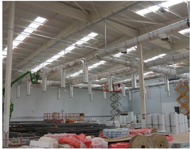
New Build Ductwork Installation Work
