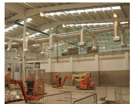
Aluminium Ductwork Installation
