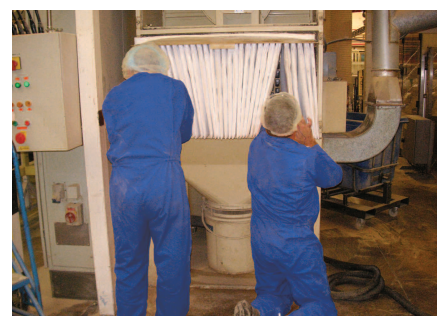
Service Work being carried out on a LEV Dust Collector
