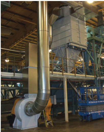
LEV System Design and Installation
