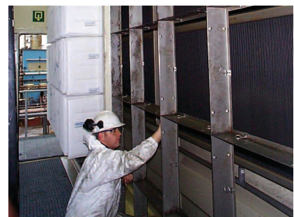
AHU Service and Maintenance
