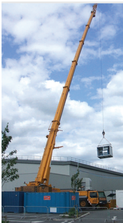
AHU Crane Lift
