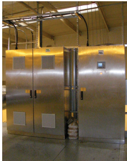
Integrated Ventilation System Control Panel
